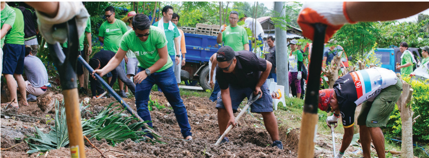
Lexmarkers installing the Gawad Kalinga rainwater catchment system in Cebu, Philippines
