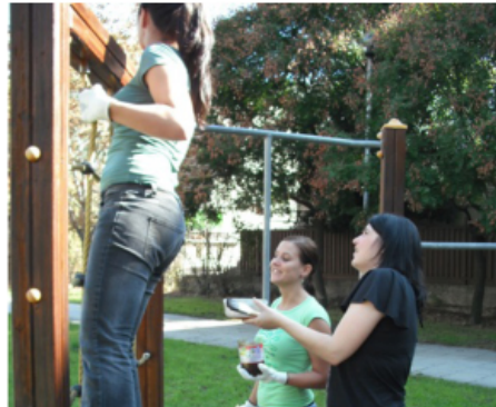
Kindergarten painting and renovation
